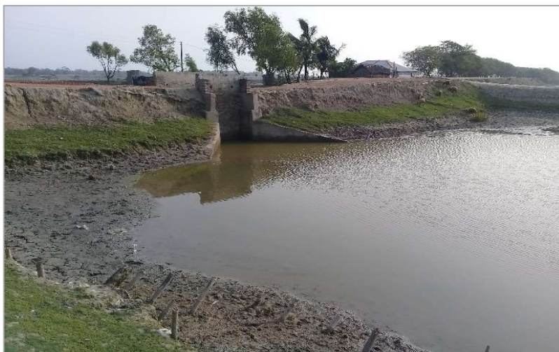
Figure_Apx 50: Polder 10-12 at Baintala Gate, Paikgacha, Khulna
