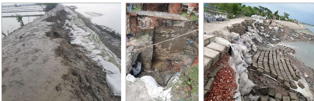
Figure_Apx 51: Embankment failure in polder 13-14/2
