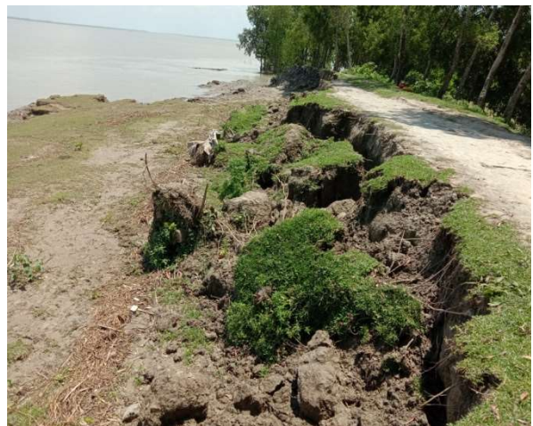
Figure_Apx 88: Polder-55/1, Location- Ratandi Taltali, Uapzilla: Galachipa , District: Patuakhali
