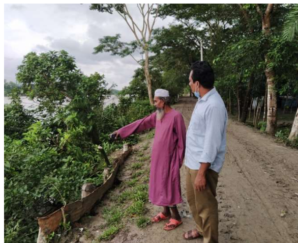
Figure_Apx 82: Polder-47.1, Location- Puran Mohipur, thana- Mohipur, Upzilla: Kalapara, Dist-Patuakhali
